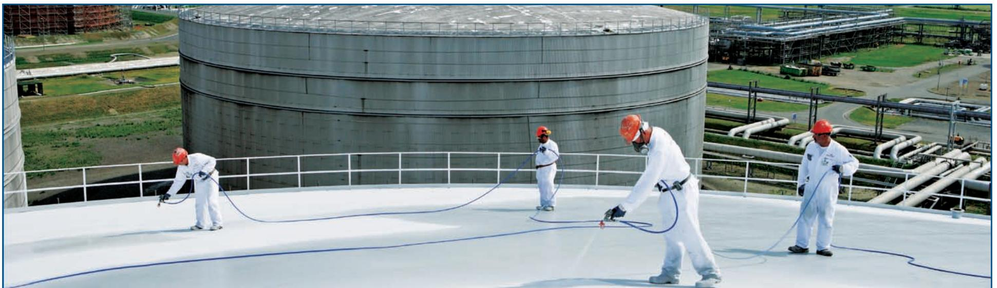
**Our thermal insulating and anti-condensation spray-applied coatings have revolutionized the way companies insulate and protect surfaces.**
